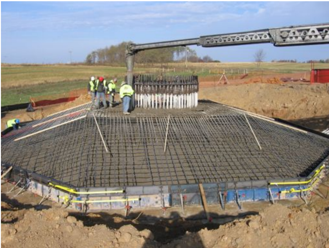
Cashton North Turbine Foundation Concrete Pour- Fall 2011
