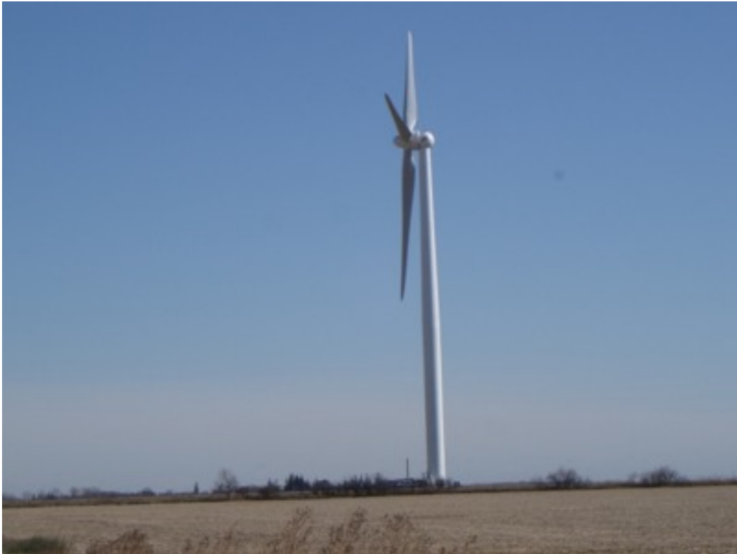
Buffalo Center Wind Turbine installed in Fall 2011
