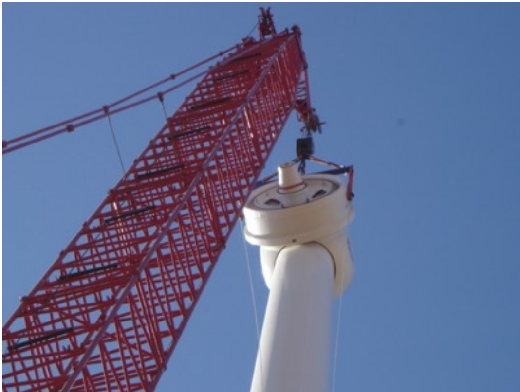
Crane installing the compact generator unit of the Goldwind 1.5MW turbine
