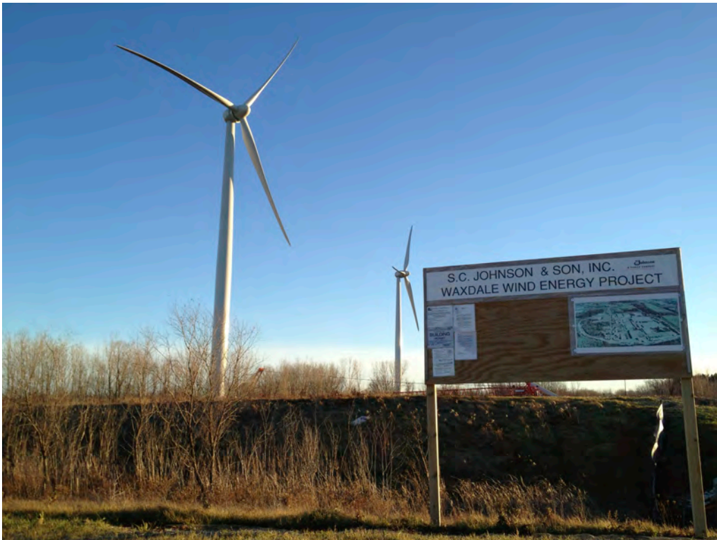
Waxdale turbines erected December 2012
